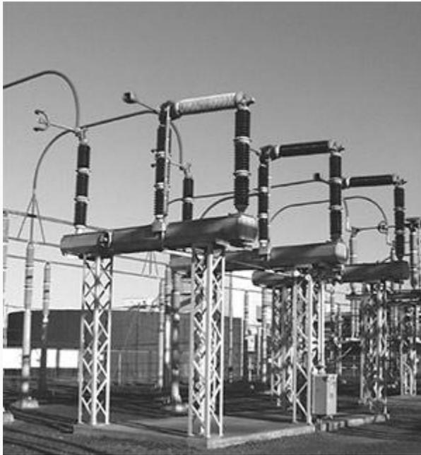
Figure 1 - Multiple interrupter gap per phase circuit switcher
