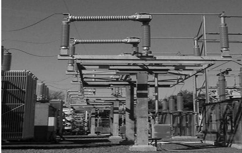
Figure 3 - Horizontal interrupter circuit switcher with integral vertical break disconnect switch.
