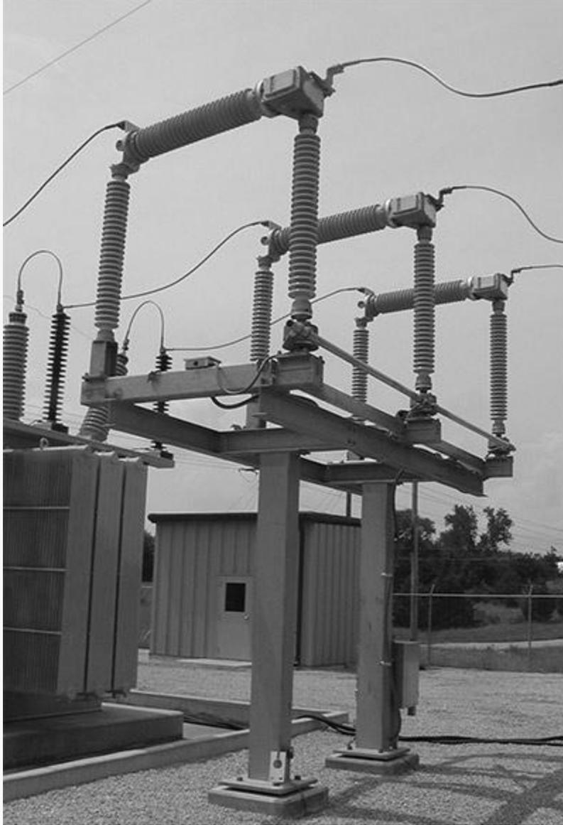
Figure 4 - Horizontal interrupter circuit switcher without integral disconnect switch
