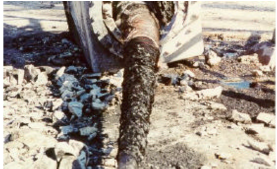
Fig 2: Failed Current Transformer
