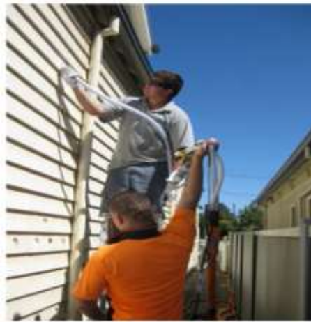
FIGURE 3.2 Injection Foam Insulation. [R. Keech]
