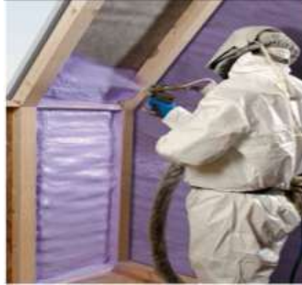
FIGURE 3.3 Spray Foam Insulation.
