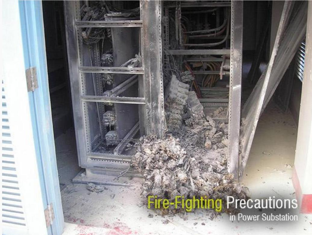
*The heat from failed capacitor bank completely destroyed the attached main incomer 400 volt switchboard for a very large shopping mall and spread the fire around substation. The radiant heat from this fire also destroyed the control panel and switchboard for the emergency power generator that was located directly opposite.*
