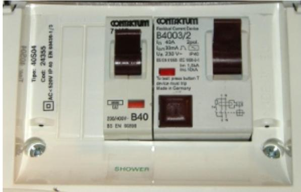
RCDs (Residual Current Devices) and can provide an element of protection against electrical shocks by disconnecting the supply if it detects a fault or if someone is having an electrical shock. RCDs are now included in domestic house wirings in the UK, but many houses were built before this regulation came into force.
