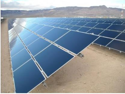
Standard solar panel ground mounts uses a framework of stainless or galvanized steel or lightweight aluminum arranged in a grid shape. The framework tilts the solar panels up toward the sun, and the angle can be either fixed or adjustable. This type of mounts requires ground surface preparation and soil testing.
