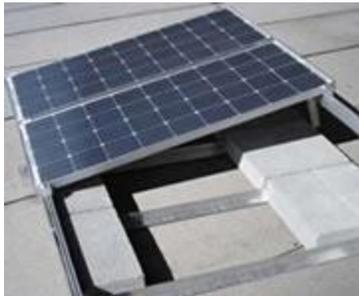
This type of mount does not require roof or soil penetration. This essentially involves a structure or frame that is held immobile by weight of concrete blocks sitting in ballast trays of the structure. To increase the friction and to protect the surface, EPDM rubber is used on the underside of the frame. The construction is typically aluminum to reduce the weight while hardware is of stainless-steel to ensure long life.
