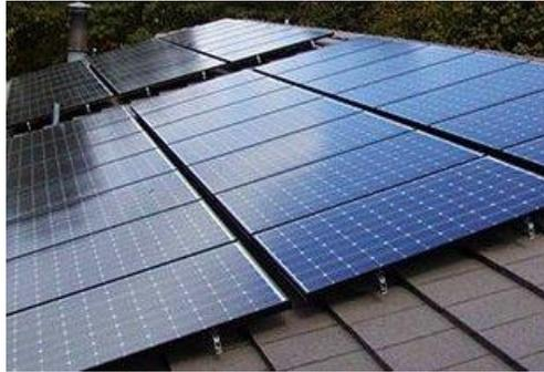
For home installations, where the weight of the panels is low, flush mounts are used. This uses a metal bracket on each side of the solar panel and holds it above the surface of the roof. There is usually at least 2-4 inches of space allowed between the panel and the roof, so that plenty of air can flow beneath the panel, and keep it cool. Overheated solar panels do not perform as efficiently and will not last long.
