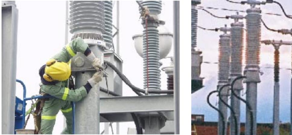
Figure 12: Installation of optical voltage and current sensors at a gas-turbine generating station.
