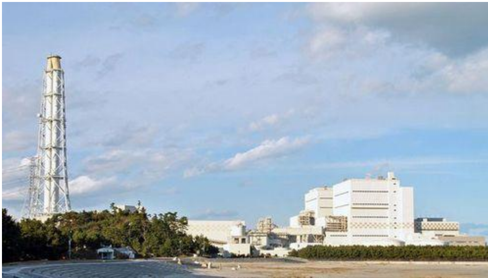
Haramachi thermal power plant
