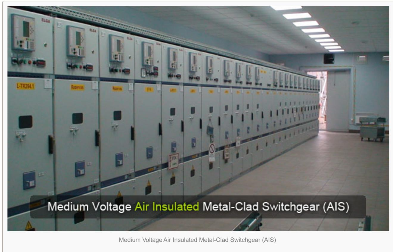
Various factors affect the reliability of a substation, one of which is the arrangement of the switching devices. Arrangement of the switching devices will impact maintenance, protection, initial substation development, and cost.
