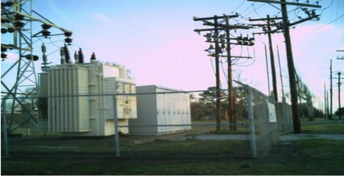
Fig 1: Primary metering with riser poles at a substation
