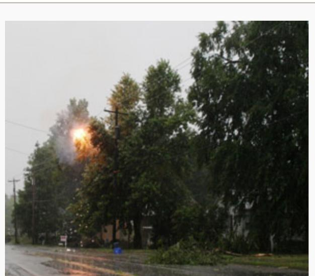
Figure 1 - Tree limbs create a short circuit during a storm, typically resulting in a power outage
