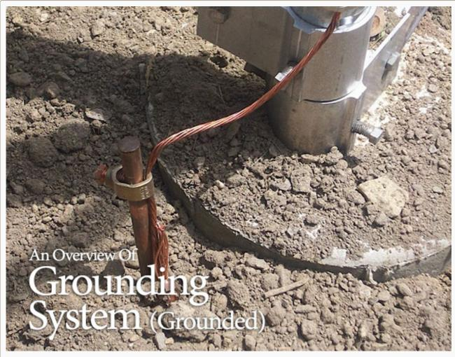
An Overview Of Grounded Grounding System (on photo: Grounded solar panel by J.E.M. Solar; jemsolar.com)
