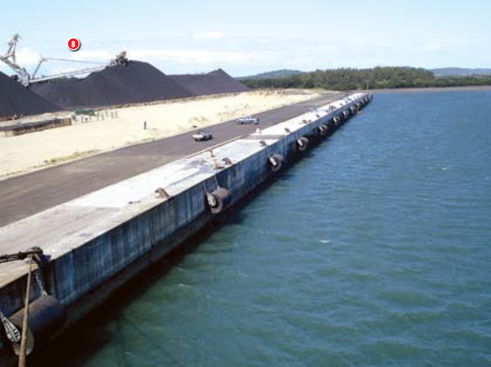
8 Completed quay wall and basin
