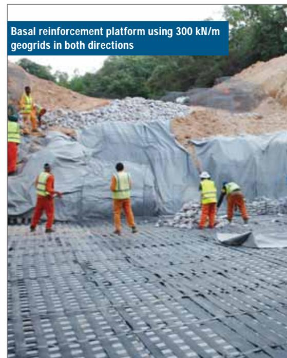
Basal reinforcement platform using 300 kN/m geogrids in both directions
