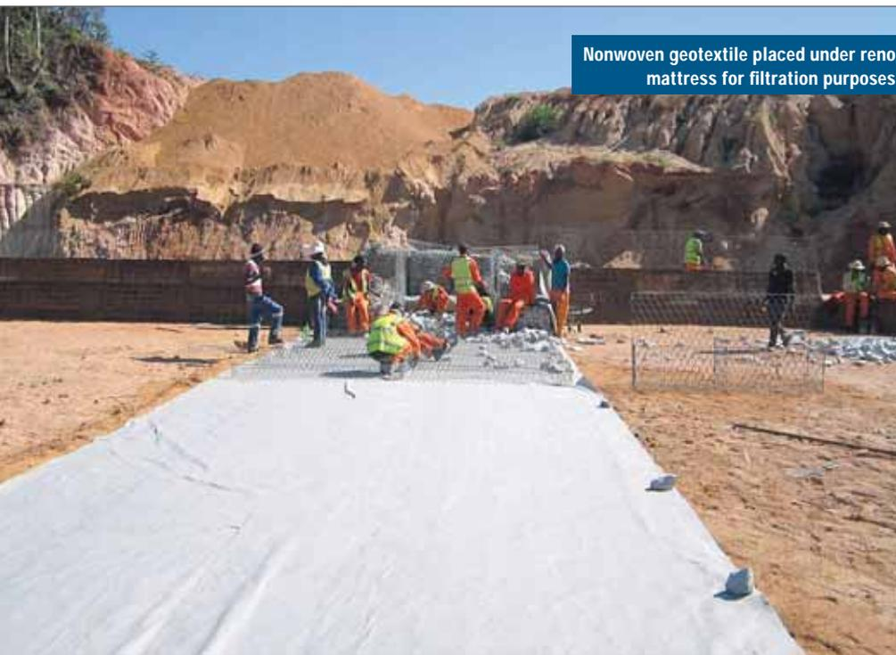
Nonwoven geotextile placed under reno mattress for filtration purposes
