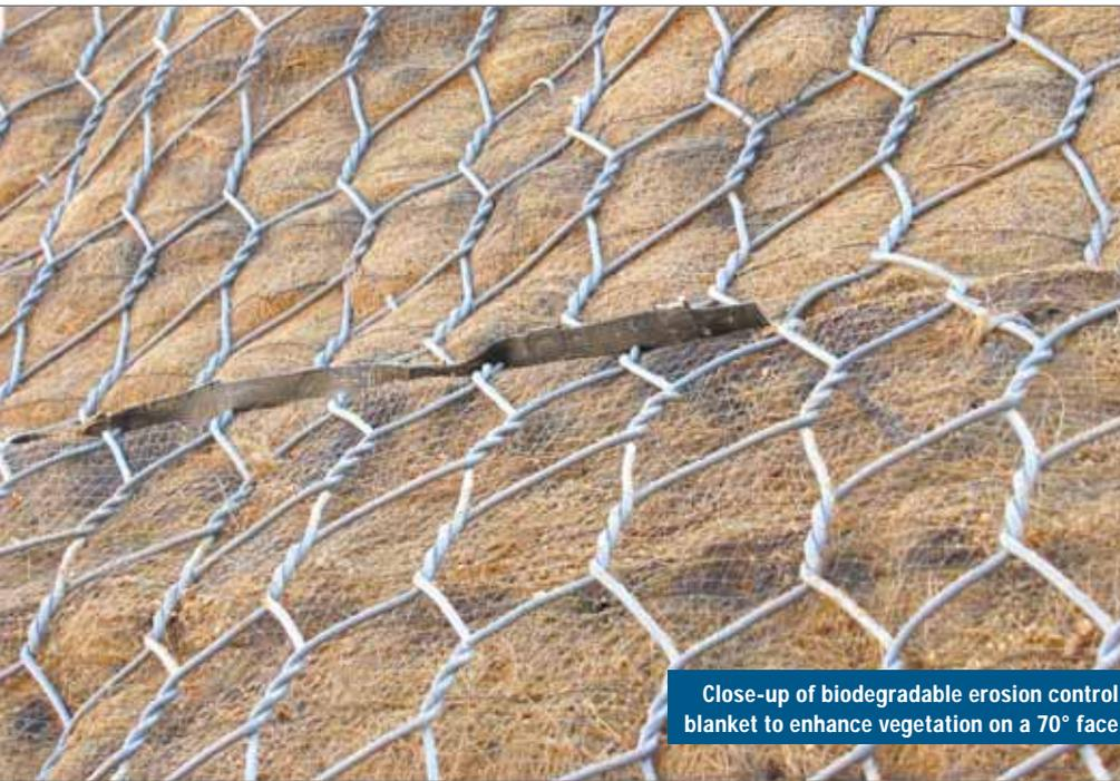
Close-up of biodegradable erosion control blanket to enhance vegetation on a 70° face
