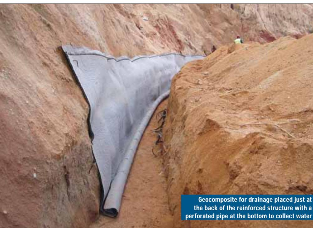
Geocomposite for drainage placed just at the back of the reinforced structure with a perforated pipe at the bottom to collect water
