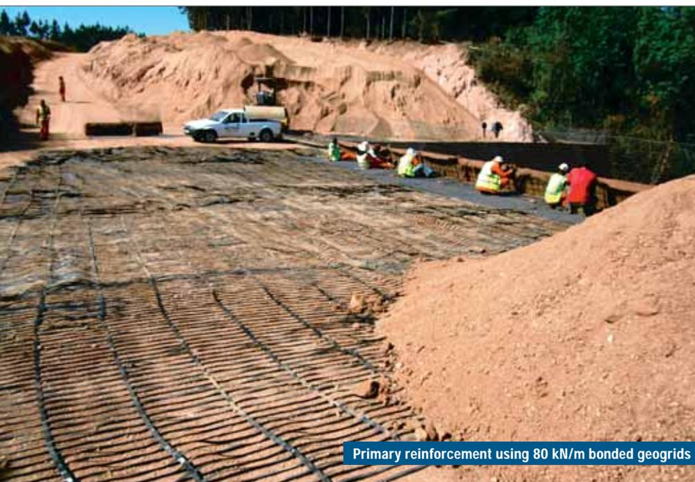
Primary reinforcement using 80 kN/m bonded geogrids
