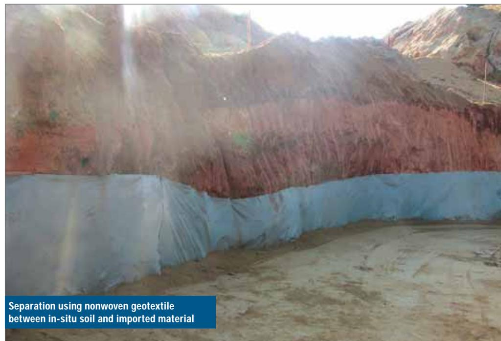
Separation using nonwoven geotextile between in-situ soil and imported material
