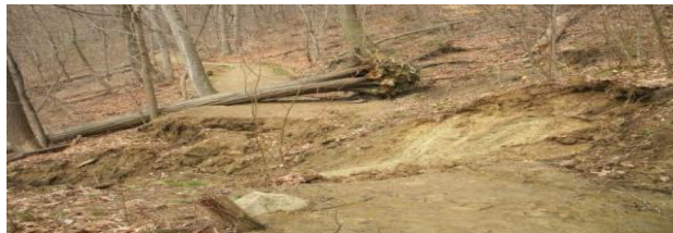
The debris flow cut out approximately 15 feet of trail. The head scarp is visible on the right.
