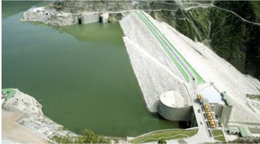
Tehri dam and reservoir (Image by Ministry of Water Resources, Government of India)
