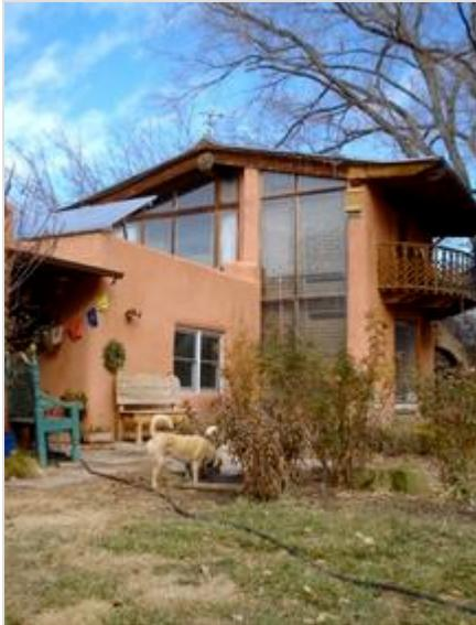
Figure 5: This home has added a two story addition which includes a Trombe wall.
