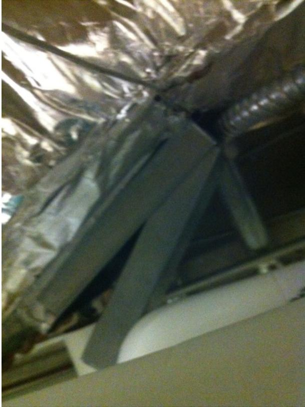
Figure 3: An access door upstream of a reheat coil blocked by piping and can't be fully opened.
