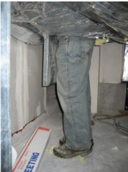
Figure 1: Good access to a smoke damper through a duct access door.
