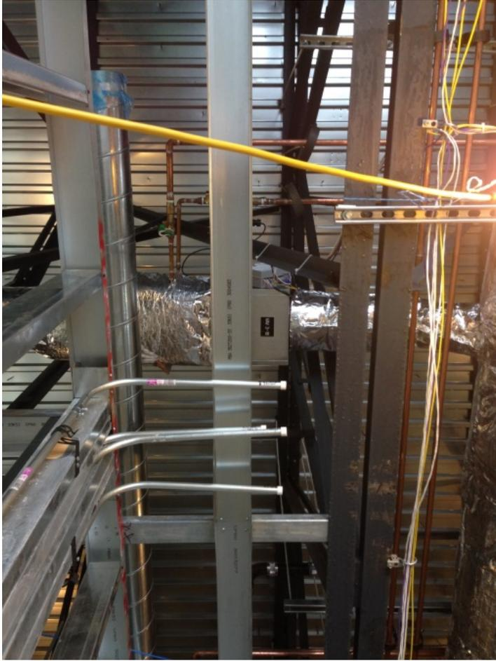
Figure 2: A VAV box blocked by a wall header and low voltage cabling.
