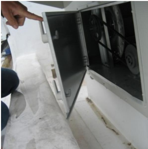
Figure 5: Access door for an RTU blocked and can't be fully opened, making service to the belt difficult.
