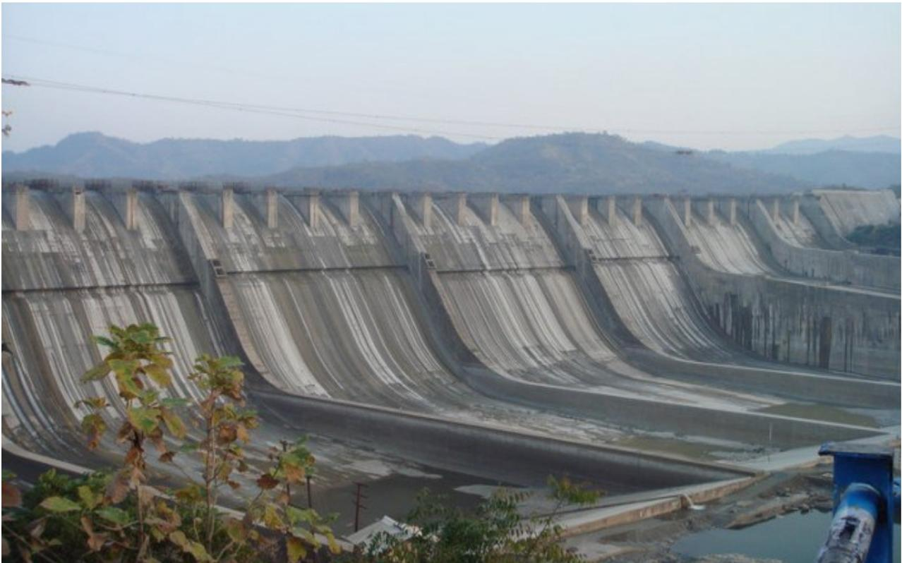
Sardar Sarovar Dam also known as “Narmada Dam” is the largest dam to be built, with a height of 163 meters, over the Sacred Narmada River in Gujarat. Drought prone areas of Kutch and Saurashtra will get irrigate by this project. The gravity dam is the largest dam of Narmada Valley Project with power facilities up to 200 MW. The dam is meant to benefit the 4 major states of India Gujarat, Madhya Pradesh, Maharashtra and Rajasthan.
