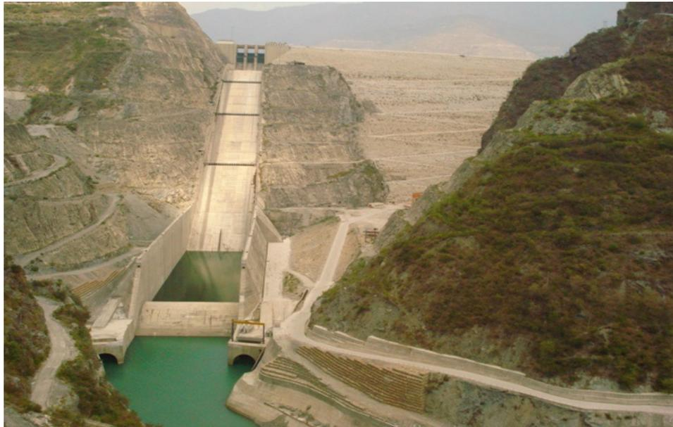
Tehri Dam located on the Bhagirathi River, Uttaranchal Now become Uttarakhand. Tehri Dam is the highest dam in India,With a height of 261 meters and the eighth tallest dam in the world. The high rock and earth-fill embankment dam first phase was completed in 2006 and other two phases are under construction. The Dam water reservoir use for irrigation, municipal water supply and the generation of 1,000 MW of hydroelectricity.
