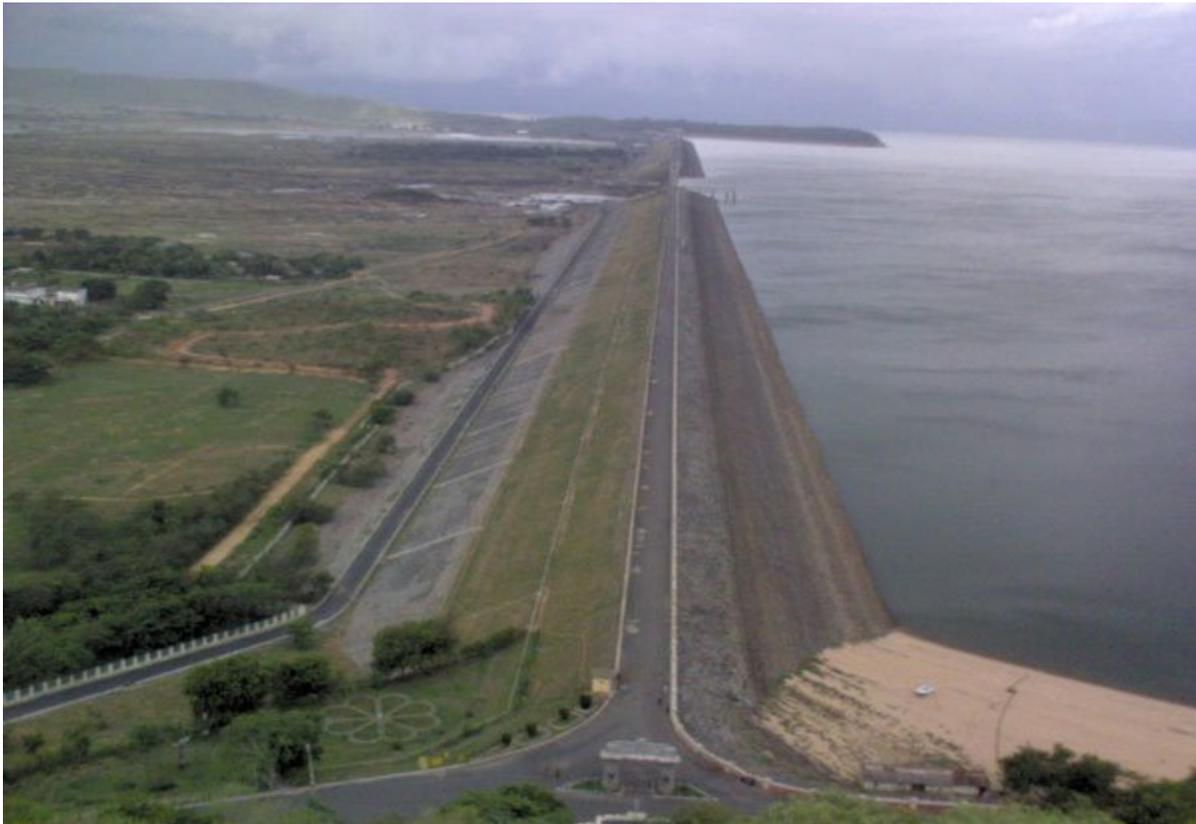
Hirakud dam built across the Mahanadi River in tribal state Orissa. Hirakud Dam is one of the longest dams in the world about 26 km in length. There are two observation towers on the dam one is “Gandhi Minar” and another one is “Nehru Minar”. The Hirakud Reservoir is 55 km long used as multipurpose scheme intended for flood control, irrigation and power generation. It was one of the major multipurpose river valley project after Independence.
