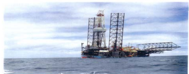
Fig. 1 a view of a drilling jack up failure due to spud can punch through (maersk drilling rig) aftert.aust
