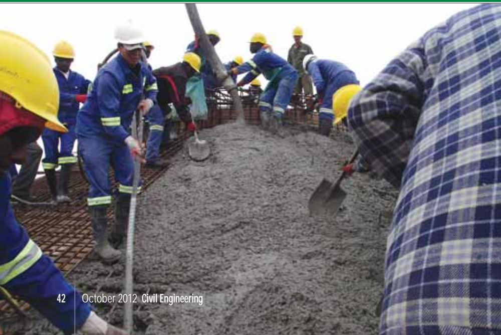
Casting the digester roof slab
