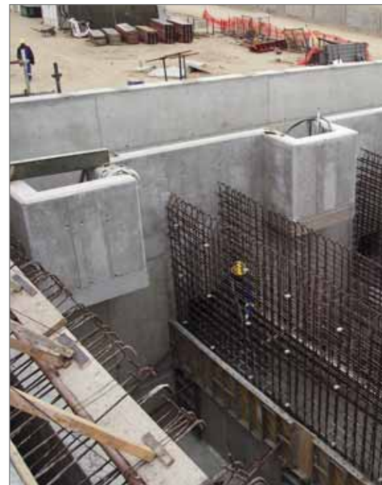
Constructing the digester
