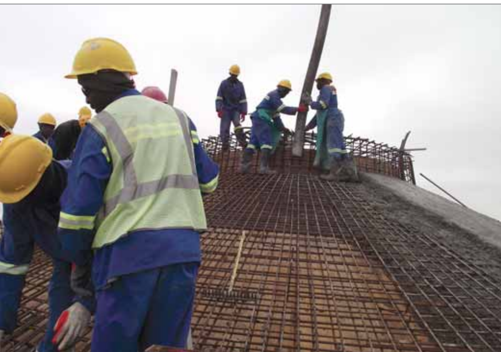
Casting the digester roof slab
