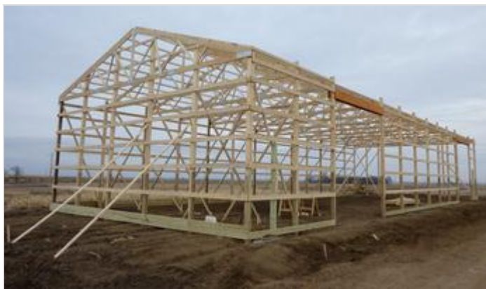
Wood truss system
