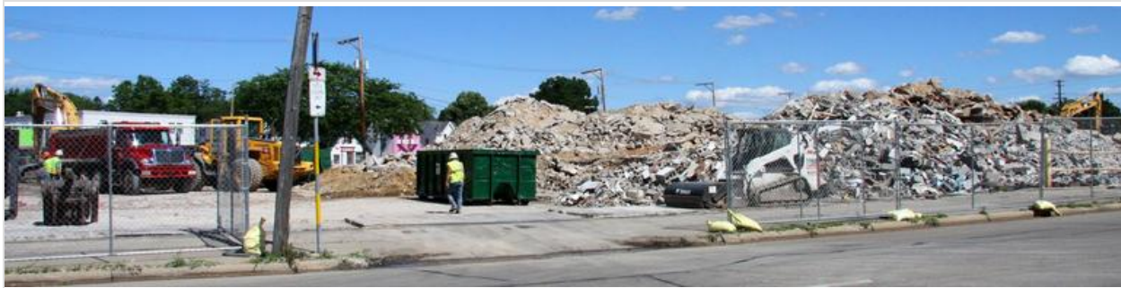
Typical site for concrete recycling
