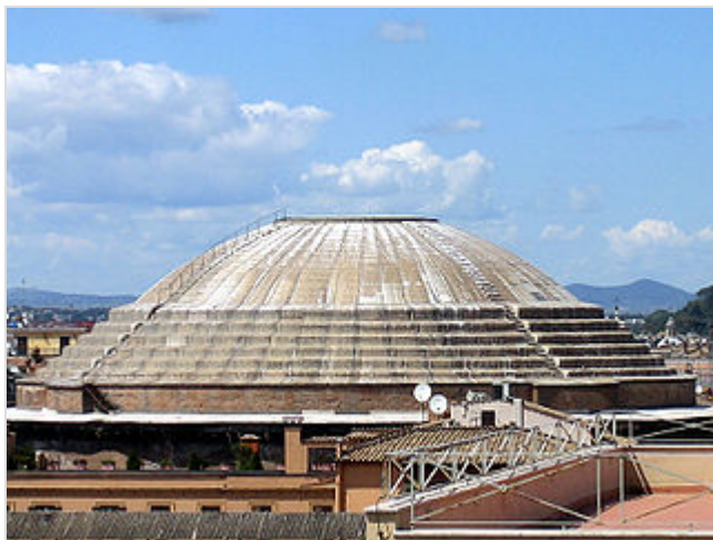
The Roman Pantheon is still the largest unreinforced solid concrete structure
