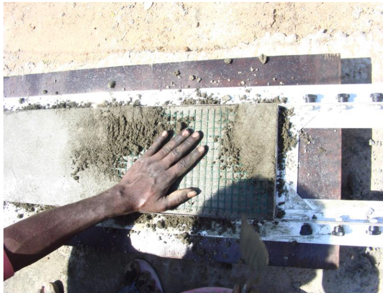
Fig. 1 Typical Casting of Ferrocement Slabs with PVC-coated Mesh
