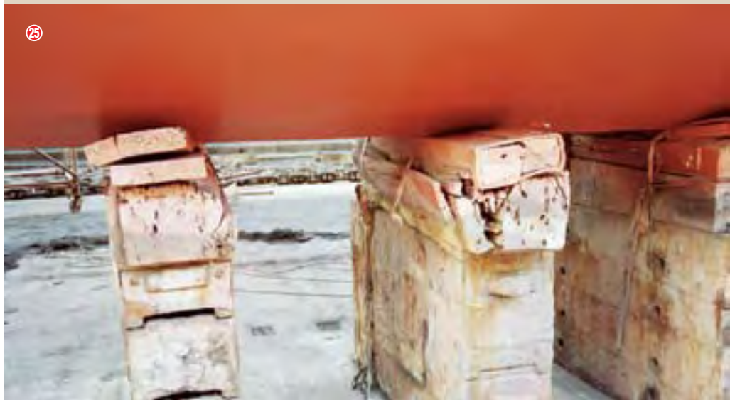
► Figure 25 Poor condition of keel blocks at the Sturrock Dock
