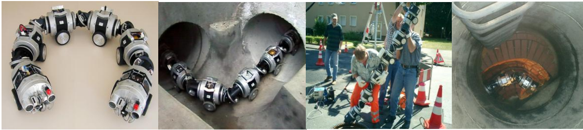
Fig. 6 The service robot MARKO plus during the examination of the rainfall canals
