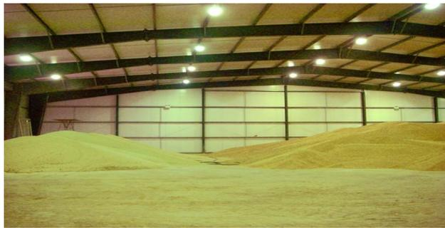
*A lightweight insulated shed raised over a massive, uninsulated floor resting on the subsoil.*
