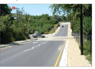
A significant challenge that the team faced on site, for example, was the construction of the pavement layers through the town of Pniel by means of in-situ recycling. The road reserve was narrow and, in many instances the existing houses, many of which were old and of historic significance, were built on the reserve edge. The contractor therefore had to ensure that all the necessary precautions were in place in order to mitigate any damage to the structures as a result of the recycling
