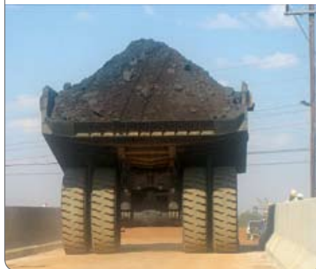
Figure 5 The completed bridge in operation
