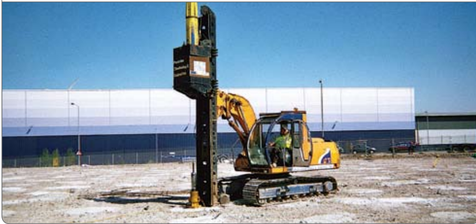
Figure 1 Equipment for the 'rapid' pile test up to 1 500 kN
