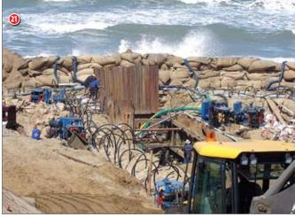
Excavation and dewatering for landline beach connection under way.
