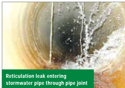
Burst pipe located during investigation in Wells Estate
