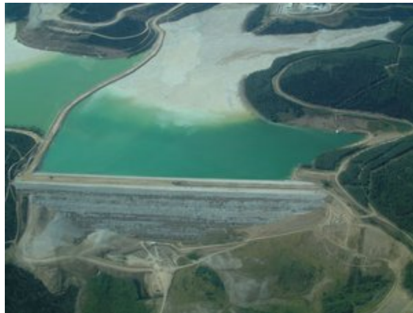
Earthen tailings impoundment dam at Fort Knox gold mine in Alaska
