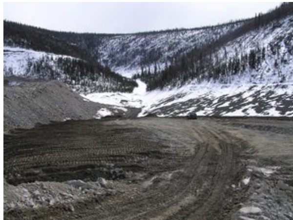
Pogo Mine Tailings Facility
