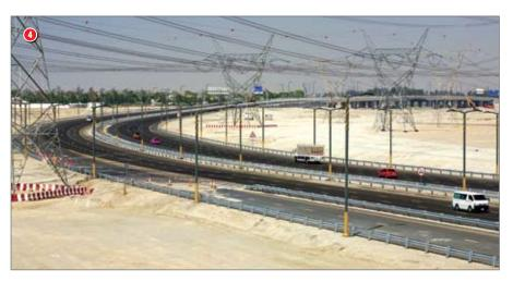
carrying Meydan Road over the canal. All the bridges were constructed as posttensioned concrete box girders.
