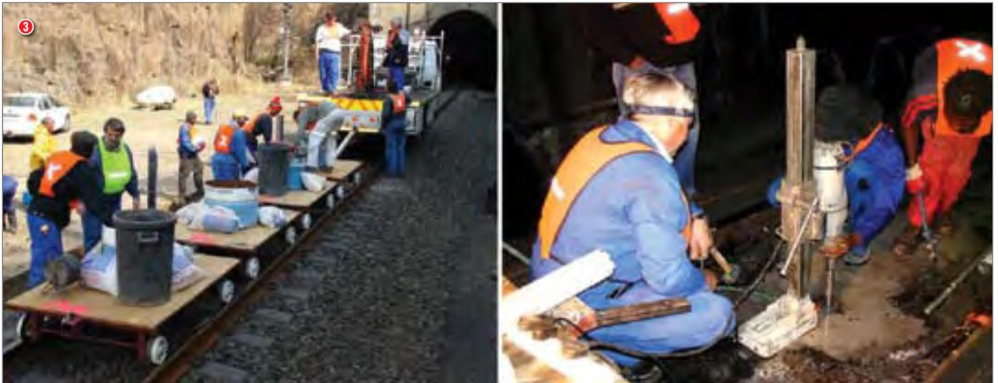
► **Figure 3** The core drilling investigation with three purpose-built trolleys combined to form an investigation 'train'
