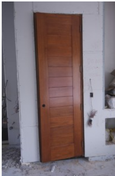
The wine cellar door
