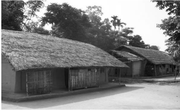
Fig.7 The front to the house
