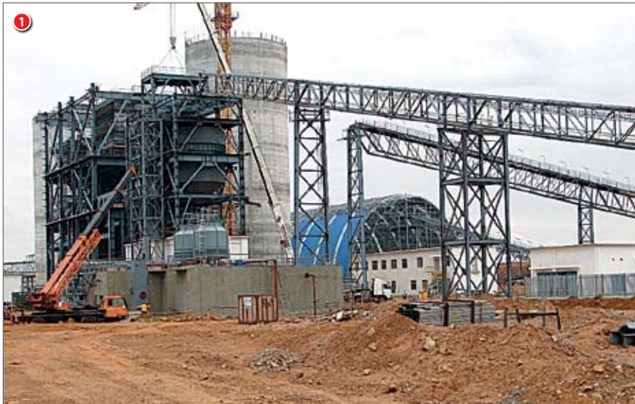
1 Lafarge's Randfontein grinding plant under construction
