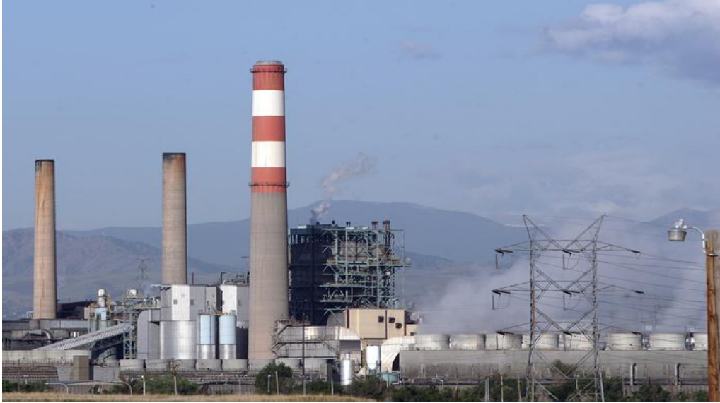
An industrial park smoke stack in Denver, Colorado
