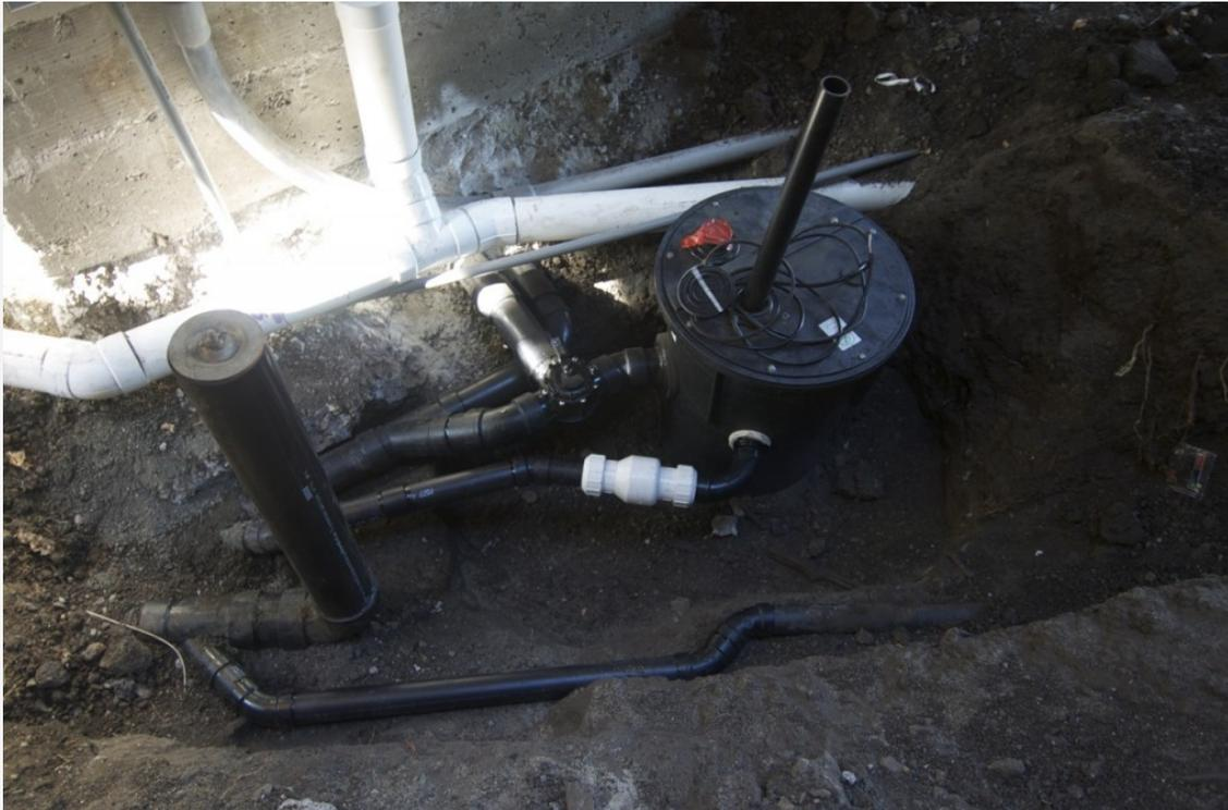
The grey water outlet showing the diverter valve, surge tank with top discharge, overflow line with check valve and all the exits to the main sewer at left
