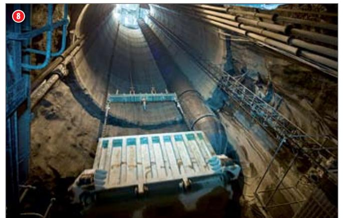
The crane is clad with sound absorbing panels to limit noise created by construction work. This is a temporary structure, which will be removed once tunnelling operations are completed.
