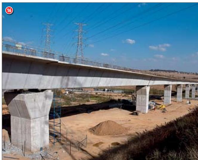
its work at Viaduct 3. Once the launching girder is assembled, deck erection will commence.
