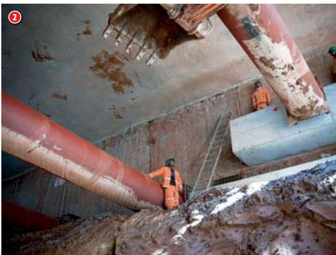
Within the station box, waler beams and struts have been installed to provide temporary lateral support to the perimeter walls during station box excavation.
