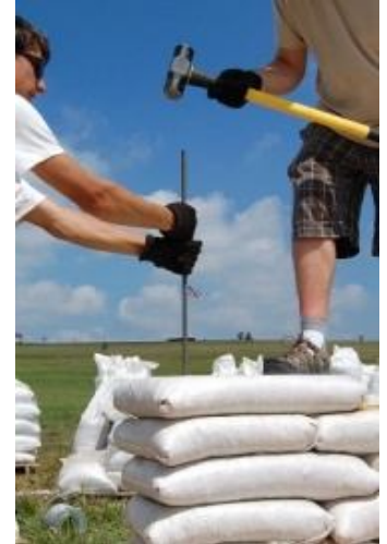
Right: Hammering vertical rebar into earthbags
