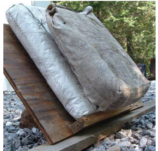
Above: The top earthbag is held up by barbed wire alone
