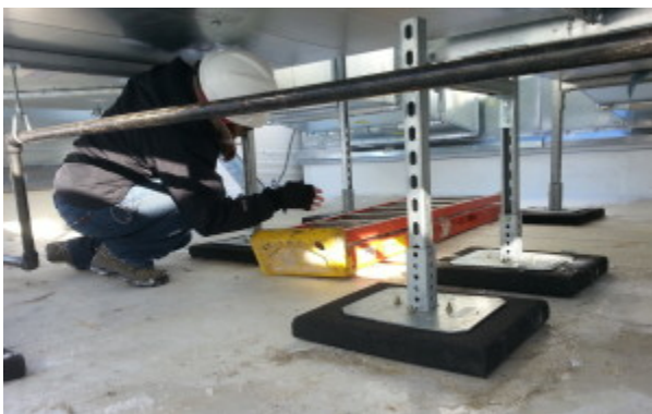
A commissioning engineer inspects duct work.
