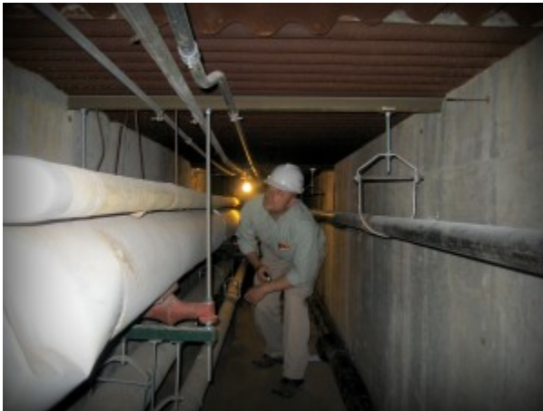
A commissioning agent inspects piping
