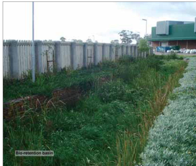
A similar stormwater bio-swale as this one at the Kraaifontein Waste Management Centre in Cape Town will be built at the Electron Road site
