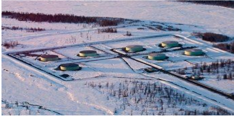
Storage tanks for oil
