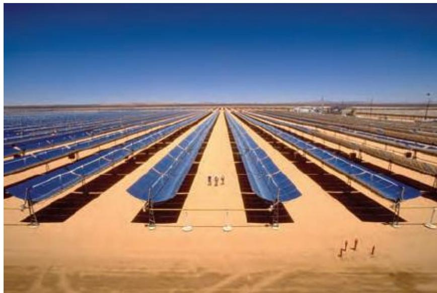
Large desert-based power plants concentrate the sun's energy to produce high-temperature heat for industrial processes or to convert the solar energy into electricity. It is quite interesting to note that, as per the recent reports on Solar Power, the resource calculations show that just seven states in the U.S. Southwest can provide more than 7 million MW of solar generating capacity, i.e., roughly 10 times that of total electricity generating capacity of U.S. today from all sources.
