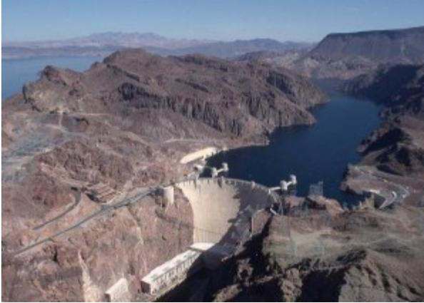
An arch dam is quite suitable for narrow canyons with strong flanks which are capable of resisting the thrust produced by the arch action. The section of an arch dam is approximately triangular like a gravity dam but the section is comparatively thinner. The arch dam may have a single curvature or double curvature in the vertical plane. Generally, the arch dams of double curvature are more economical and are used in practice.
