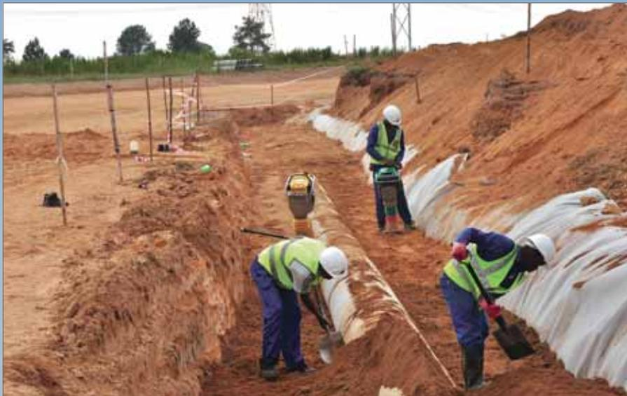
A section of 650 mm concrete piping is covered with soil after laying and joining. A layer of bidem sheeting which is installed to prevent excess water from penetrating beneath the road surface can be clearly seen
