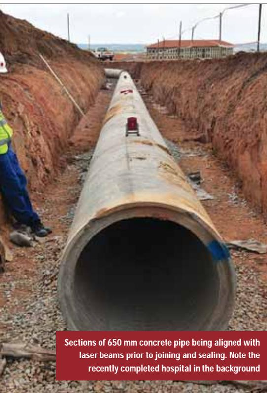
Sections of 650 mm concrete pipe being aligned with laser beams prior to joining and sealing. Note the recently completed hospital in the background
