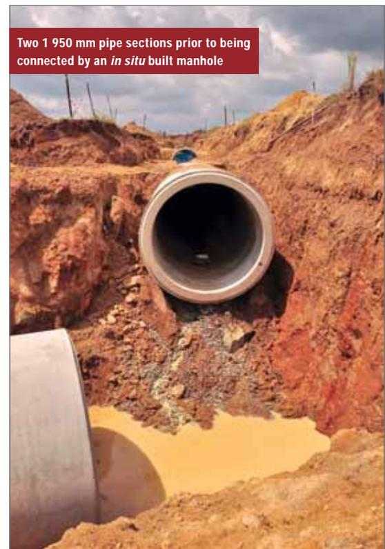
Two 1 950 mm pipe sections prior to being connected by an *in situ* built manhole
