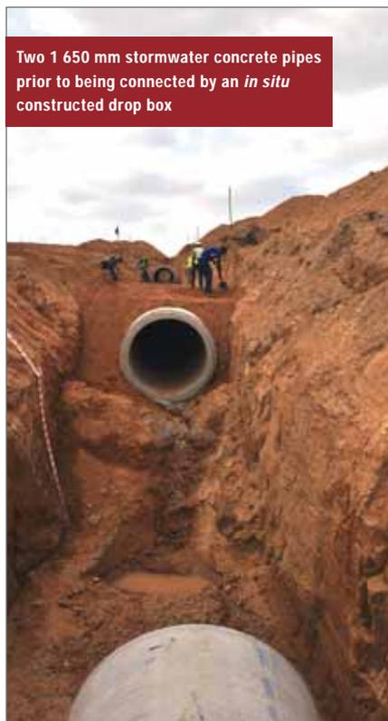
Two 1 650 mm stormwater concrete pipes prior to being connected by an *in situ* constructed drop box
