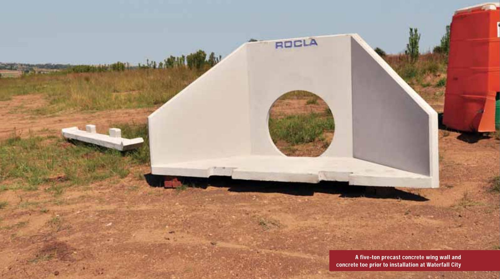
A five-ton precast concrete wing wall and concrete toe prior to installation at Waterfall City
