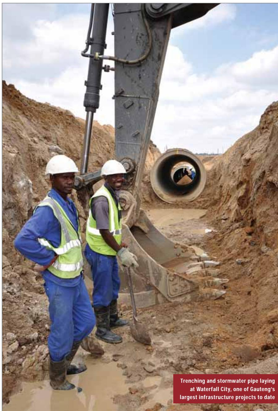
Trenching and stormwater pipe laying at Waterfall City, one of Gauteng's largest infrastructure projects to date
