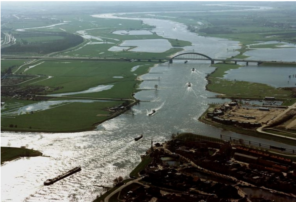
River Training Works
