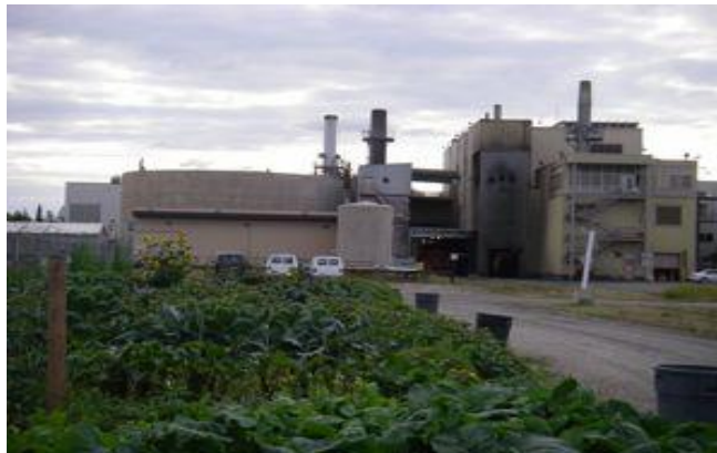
UAF power plant - photo Russ Maddox
